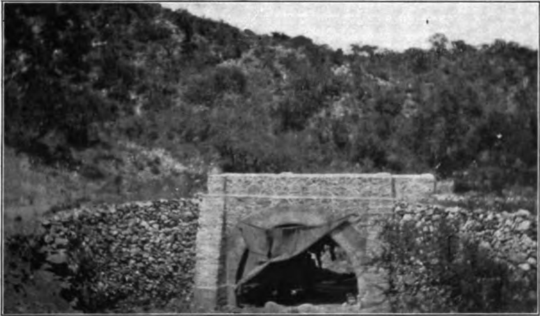
Bridge on Road to Dique San Roque
